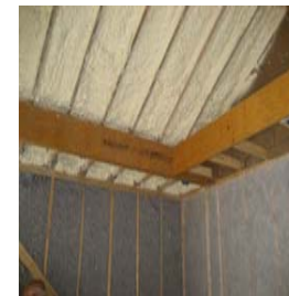
Cellulose wall assembly and a foam roof deck paired as an energy efficient system for this Building.
